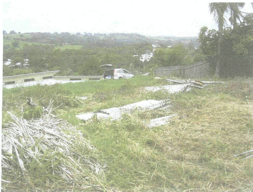
Photograph 3 Site 7 Building Rubble (Rear of site)
